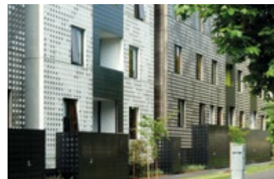
Residential building façade
